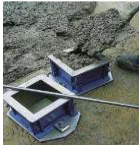
placing of concrete
